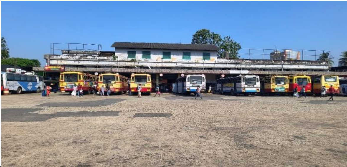
Figure 1: KSRTC Bus Terminal Thrissur
